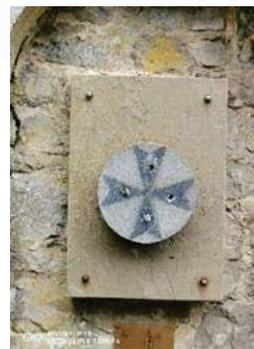
Fig. 2. Perimeter wall plate.
