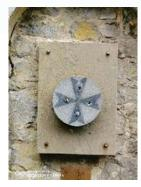
Fig. 2. Perimeter wall plate.
